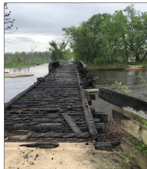
The Tank Creek Bridge on the Great River State Trail is currently closed until further notice due to damage from a fire on Thursday evening, May 15. / Photo Credit: Wisconsin DNR
